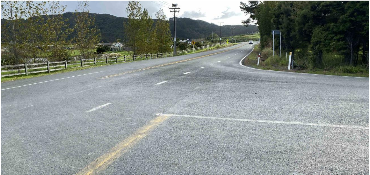
Photo 5. Looking south along Cove Road from Mangawhai Heads Road. Note the excellent visibility, the right-turn bay and the existing single-lane bridge a short distance from the intersection.
